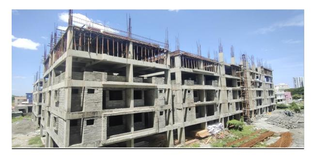
**Block A2:** Fourth Floor level slab concrete casting 100% completed. Shuttering works for 1<sup>st</sup> half of Fifth floor level slab 25% completed.
